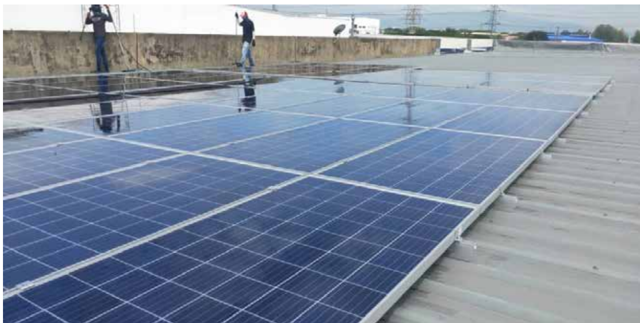
Installation of solar panel at headquarter office, Prai, Penang.
